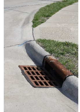
Storm drain inlet
