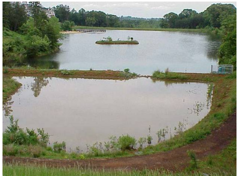
Sediment forebay at inlet of retention pond
