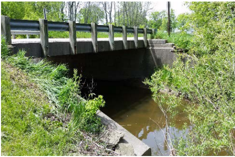
Concrete bridge All photos: MACC
