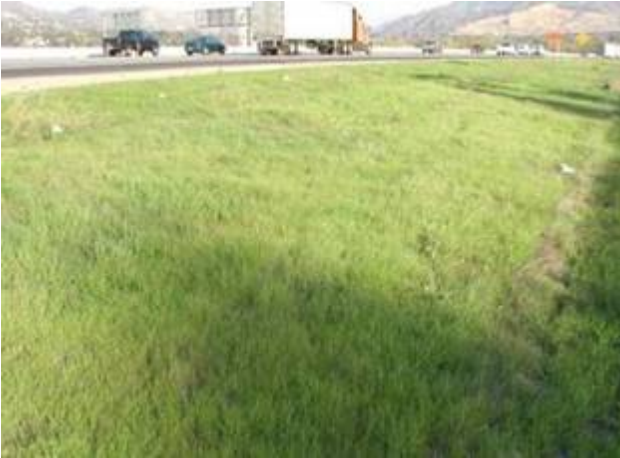
Vegetated filter strip adjacent to roadway Virginia Water Resources Research Center
