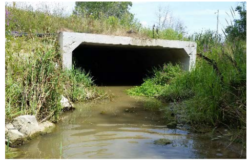
Concrete box culvert
