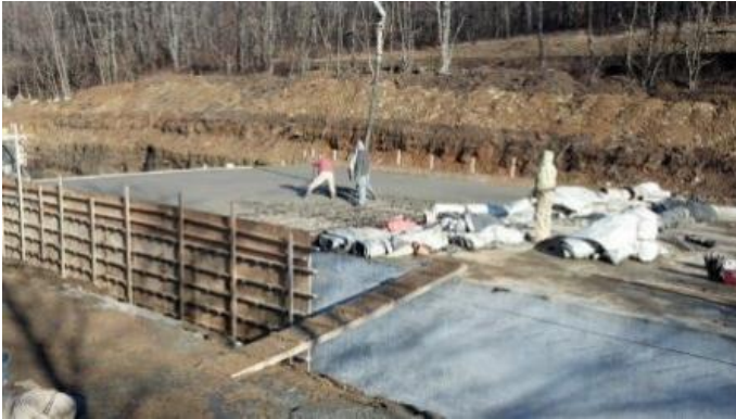
Underground cistern installation EPA
