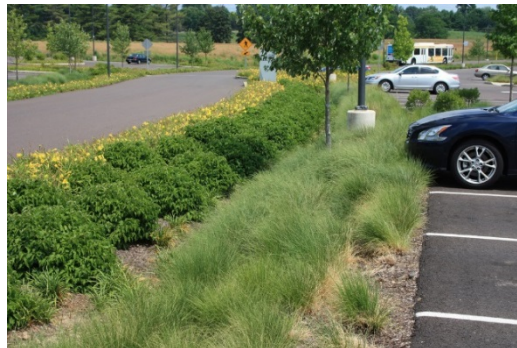
Infiltration trench, Pennsylvania Flickr
