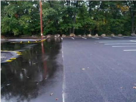
Traditional asphalt (L), permeable asphalt (R) EPA
