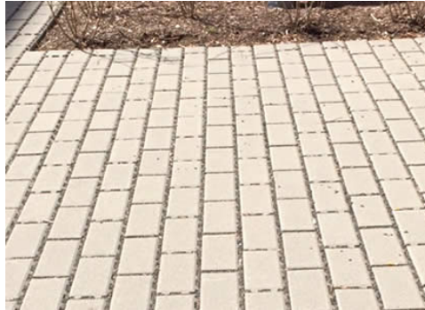
Permeable Pavers EPA
