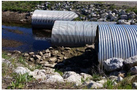
Corrugated metal culverts
