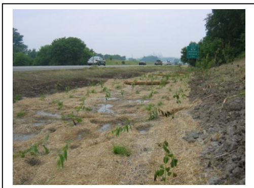
MDOT's newly constructed bioswale along West I-196
