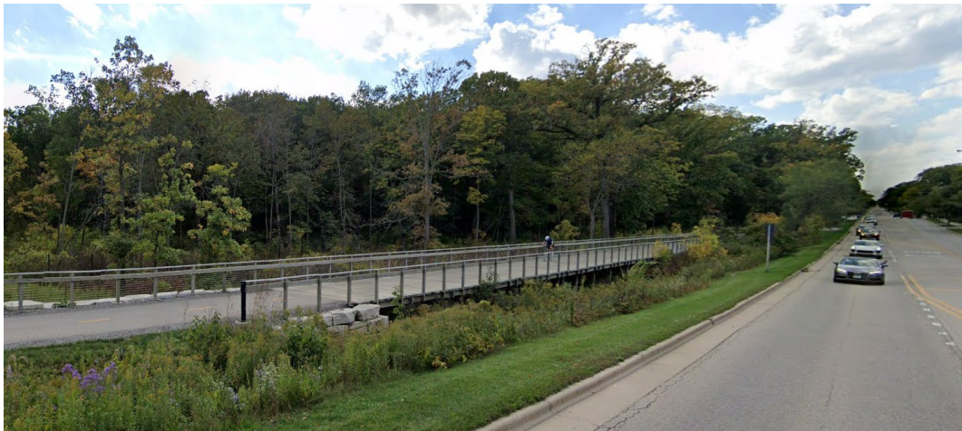
Figure 13 Example of a trail boardwalk adjacent to a road in Glencoe, IL
