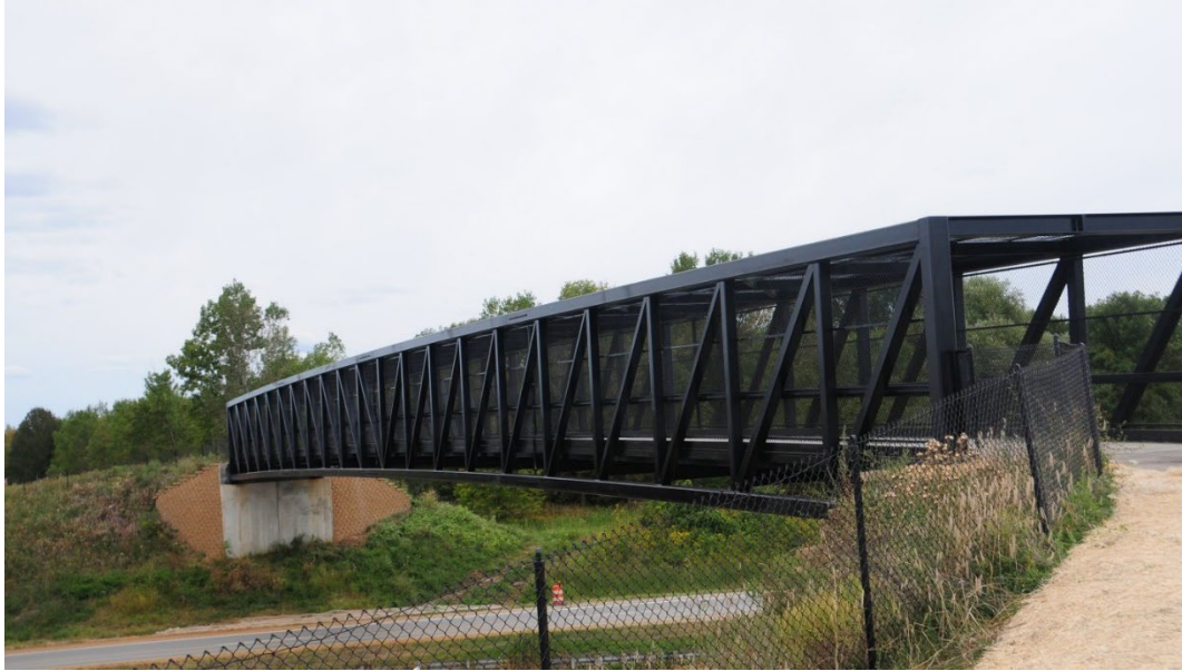
Figure 12 Example of a Pedestrian Bridge near Adams Street over I-196 in Holland Township
