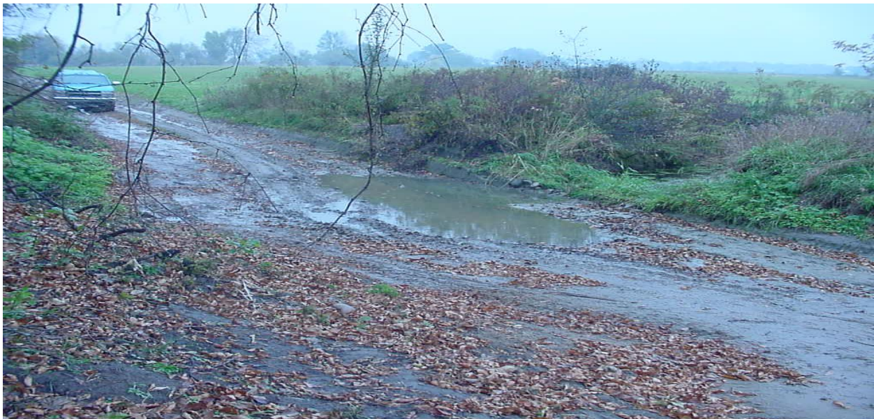
Figure 11. T- 3052, Stream Crossing (Drain Flows Over Farm Access Road)
