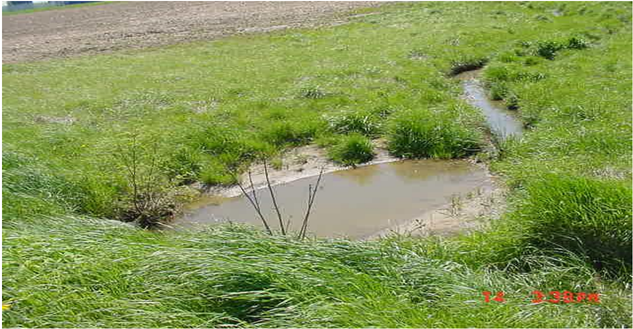
Figure 6. T – 3359, Grassed Waterway, Requires Stilling Basin (in pool) and Tile
