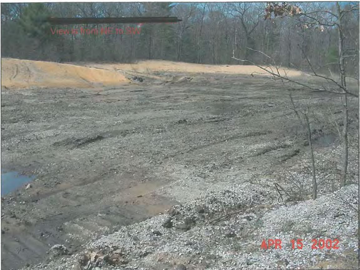
Grading at County 80 in 2002.
