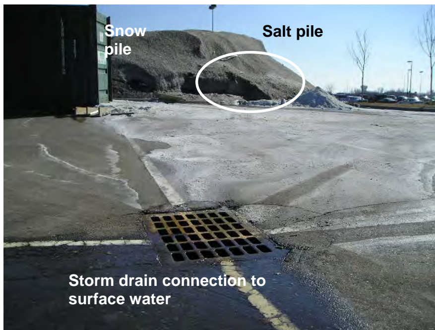
Figure 7: Incorrect salt storage: uncovered and placed in path of melting snow pile
