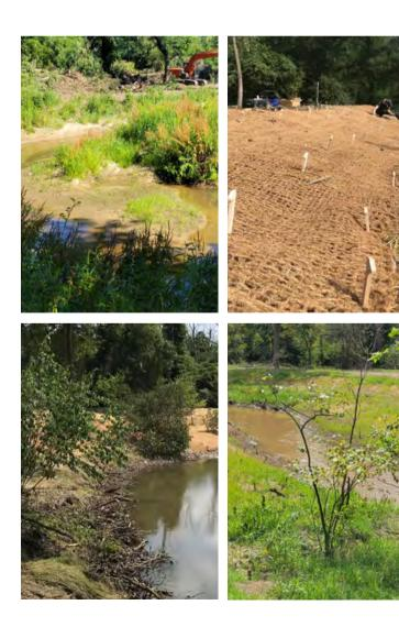
Stream and waterway restoration is another priority. Using natural stream channel design, Project Clarity restores degraded streambanks to reduce soil erosion and provide stable channels to convey water during periods of high flow. These restorations improve water quality, mitigate habitat loss to protect fish and wildlife, and protect streambanks.
