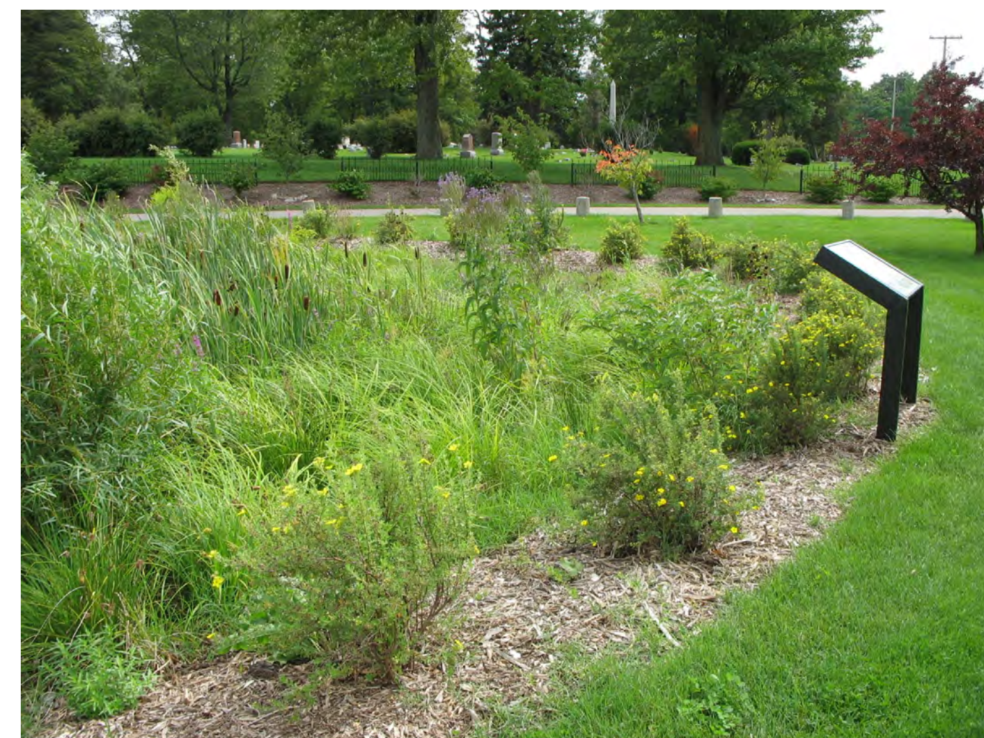
Smallenburg Park Urban Storm Water Demonstration Site (2004) A connected series of bioretention areas to encourage runoff infiltration and reduce storm water discharge from site. Streambank stabilization and wetland creation. Supported by the City of Holland, Hope College, the State of Michigan and the MACC.
