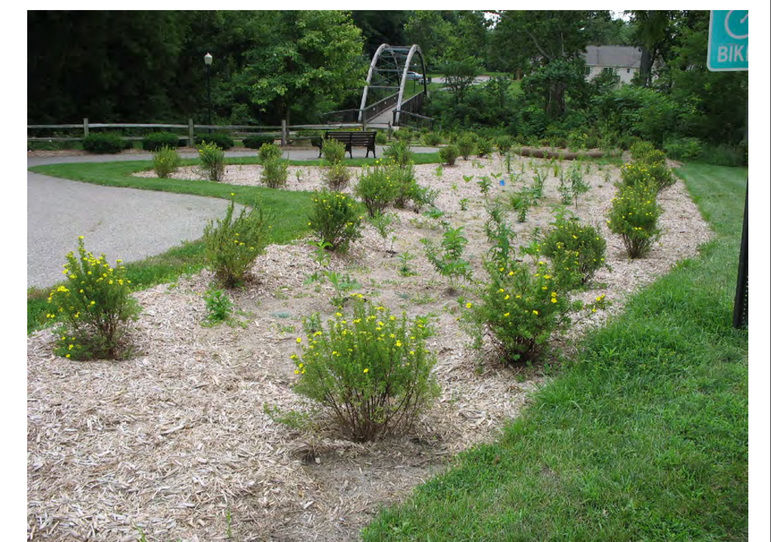
City of Zeeland Paw Paw Bridge Park Bioswale Demonstration Site (2008) Prevents erosion and treats storm water runoff from road and park via bioswale, native vegetation and increased infiltration. Supported by City of Zeeland, the State of Michigan and the MACC.
