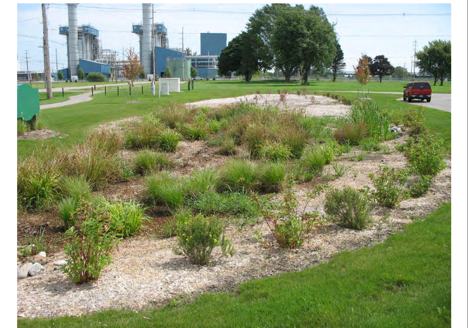
City of Zeeland Street Maintenance Facility Bioretention (2008) Replaced a typical dry detention pond with native vegetation and bioretention area. Supported by City of Zeeland, the State of Michigan and the MACC.
