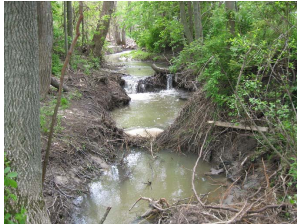
Headcut along Kuipers Drain
